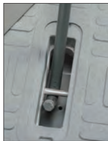
Recessed Lifting Pin with Cover
